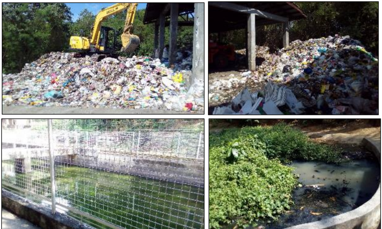
Figure 4. Material recovery facility and waste water treatment facility
